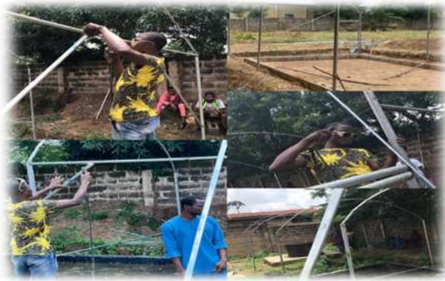
Figure 4: Welding of the aquaponics system cover steel frame
