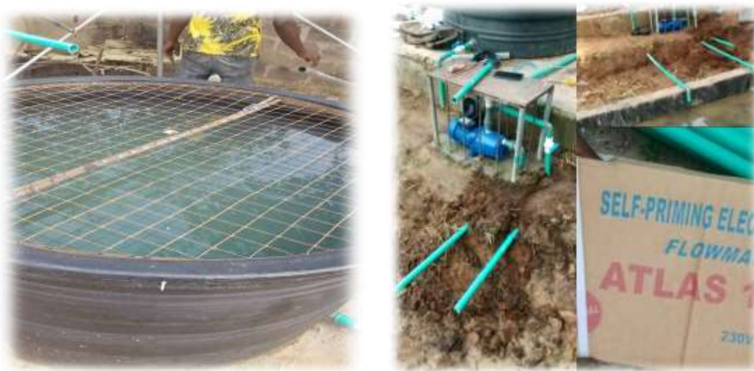
Figure 6. Pumping and Piping works for the aquaponics system
